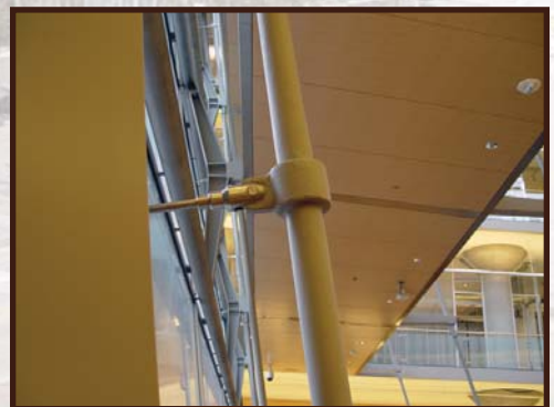
Top The completed second floor pedestrian bridge.
