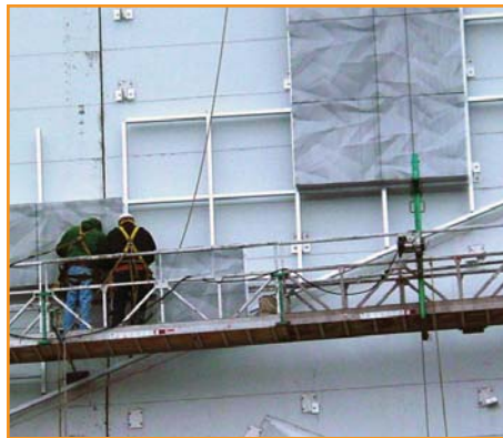
« Closer view of the paneling process. (Photo courtesy M.G. McGrath)
